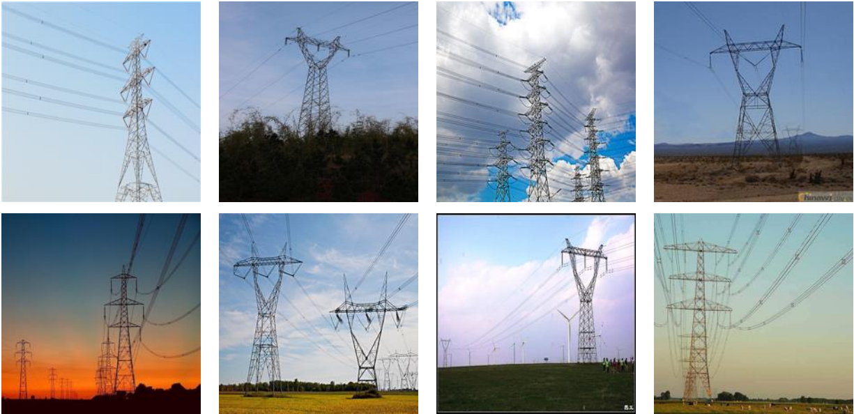
(a) Undamaged state indicating no failure
